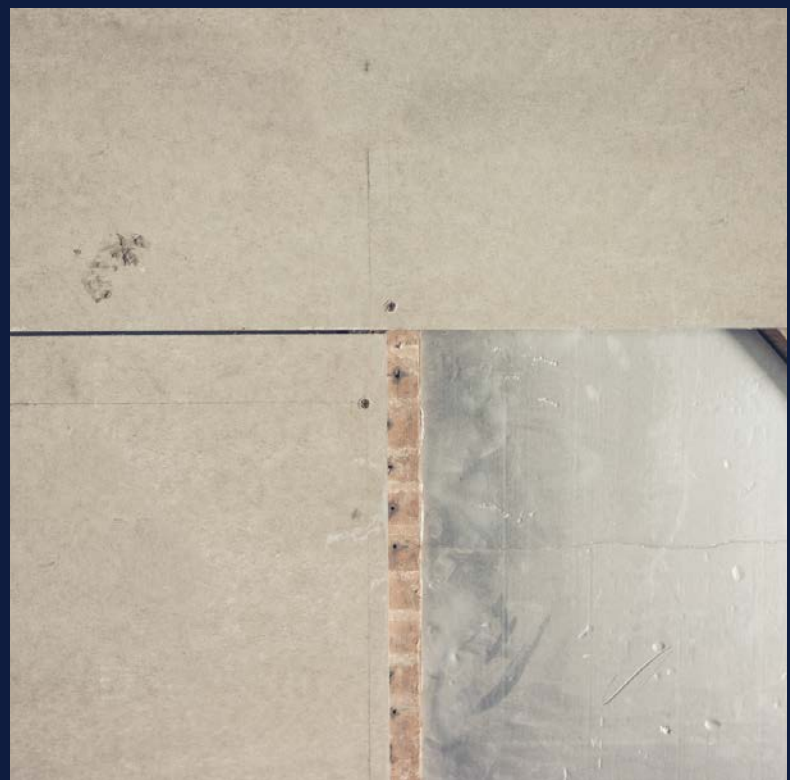
Cement board & Concrete floor deck
